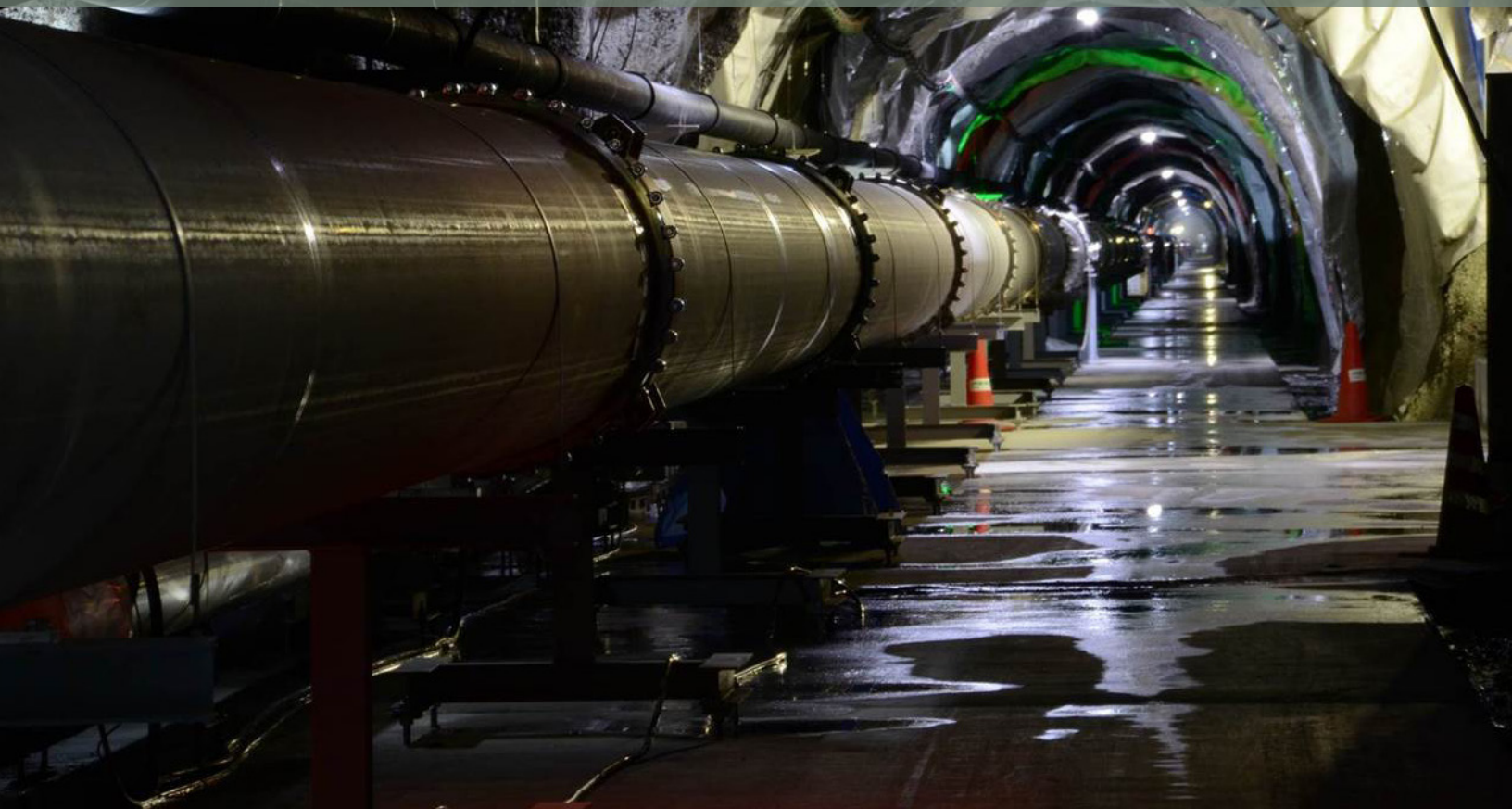
▲ KAGRA's Y-arm under construction
